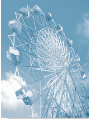
The design of members used for amusement park rides requires careful consideration of cyclic loadings that can cause fatigue.
