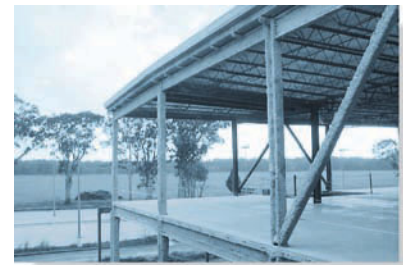
Steel rapidly loses its strength when heated. For this reason engineers often require main structural members to be insulated in case of fire.
