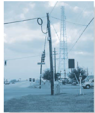
The long-term application of the cable loading on this pole has caused the pole to deform due to creep.
